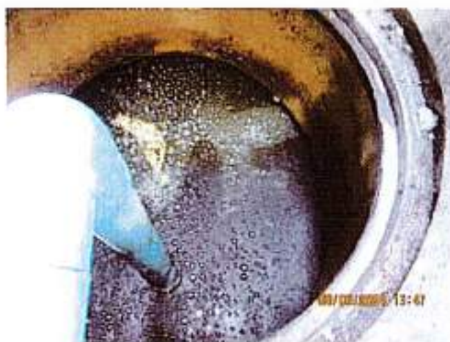
Aeration Tank 1 : No Mixing – OFF Air Blower
